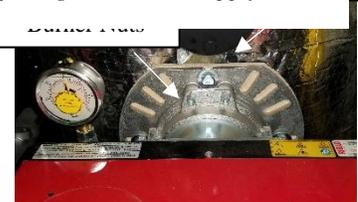
Figure 26 - Riello Burner Tube & Mounting Bracket
